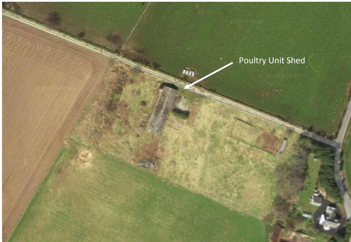
Figure 1. Poultry Unit Shed, Little Clinterty
