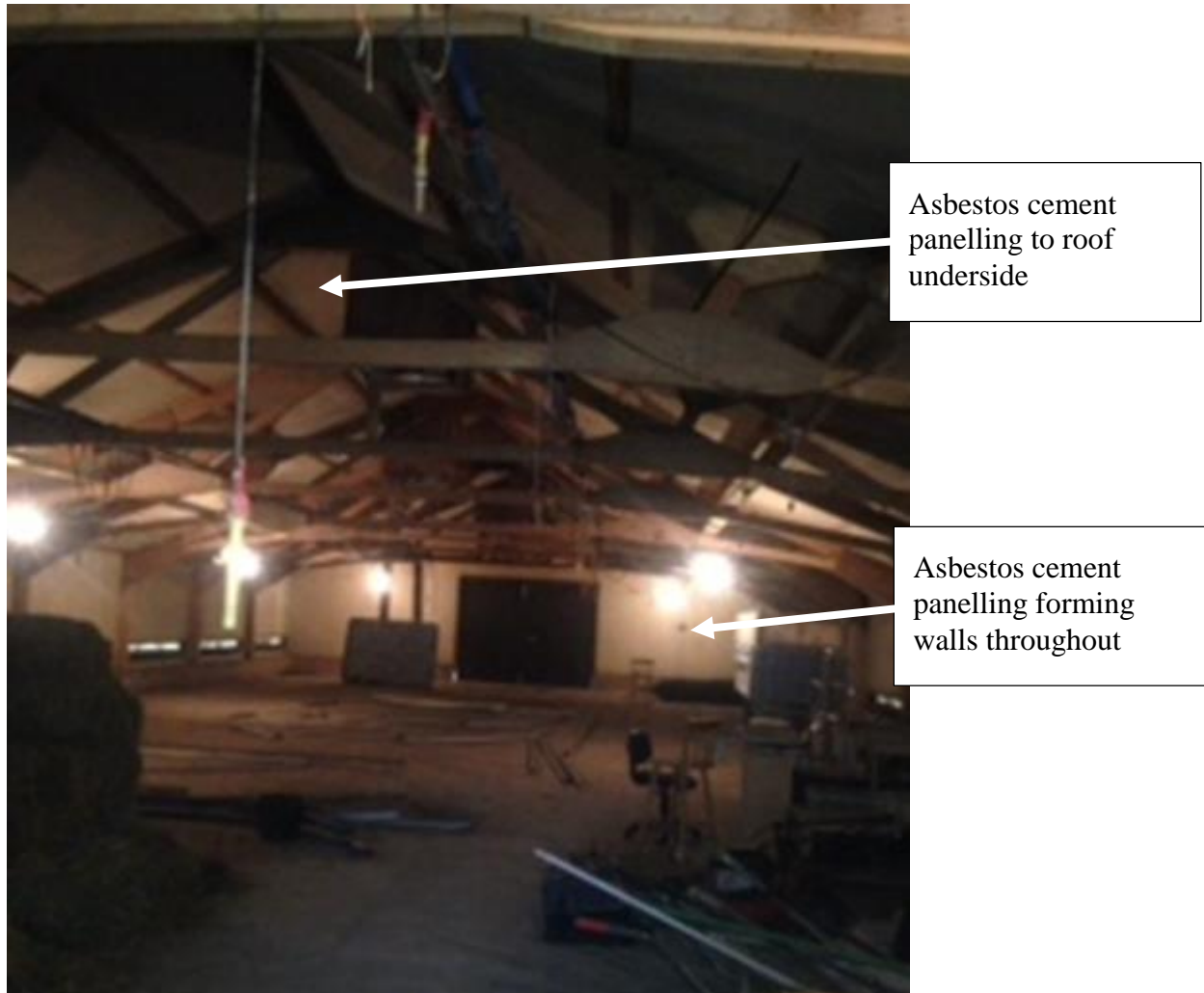
Figure 4. Internal view of barn looking south from entrance
