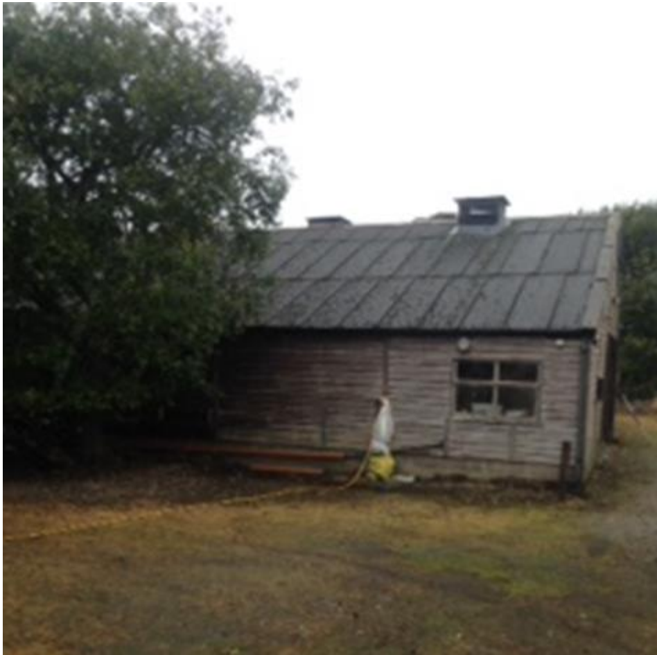
Figure 3. North (front) end of barn, east elevation
